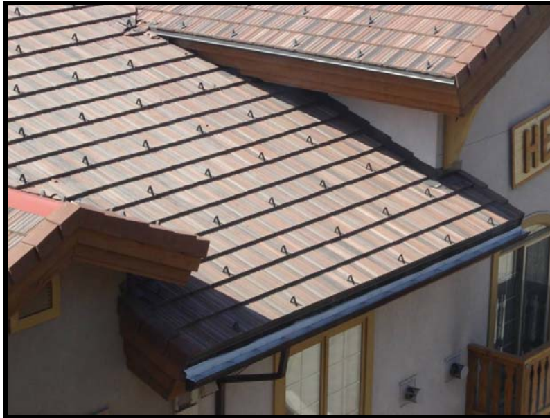
Roof Surface and Snow Clips – Village at Sun Peaks
